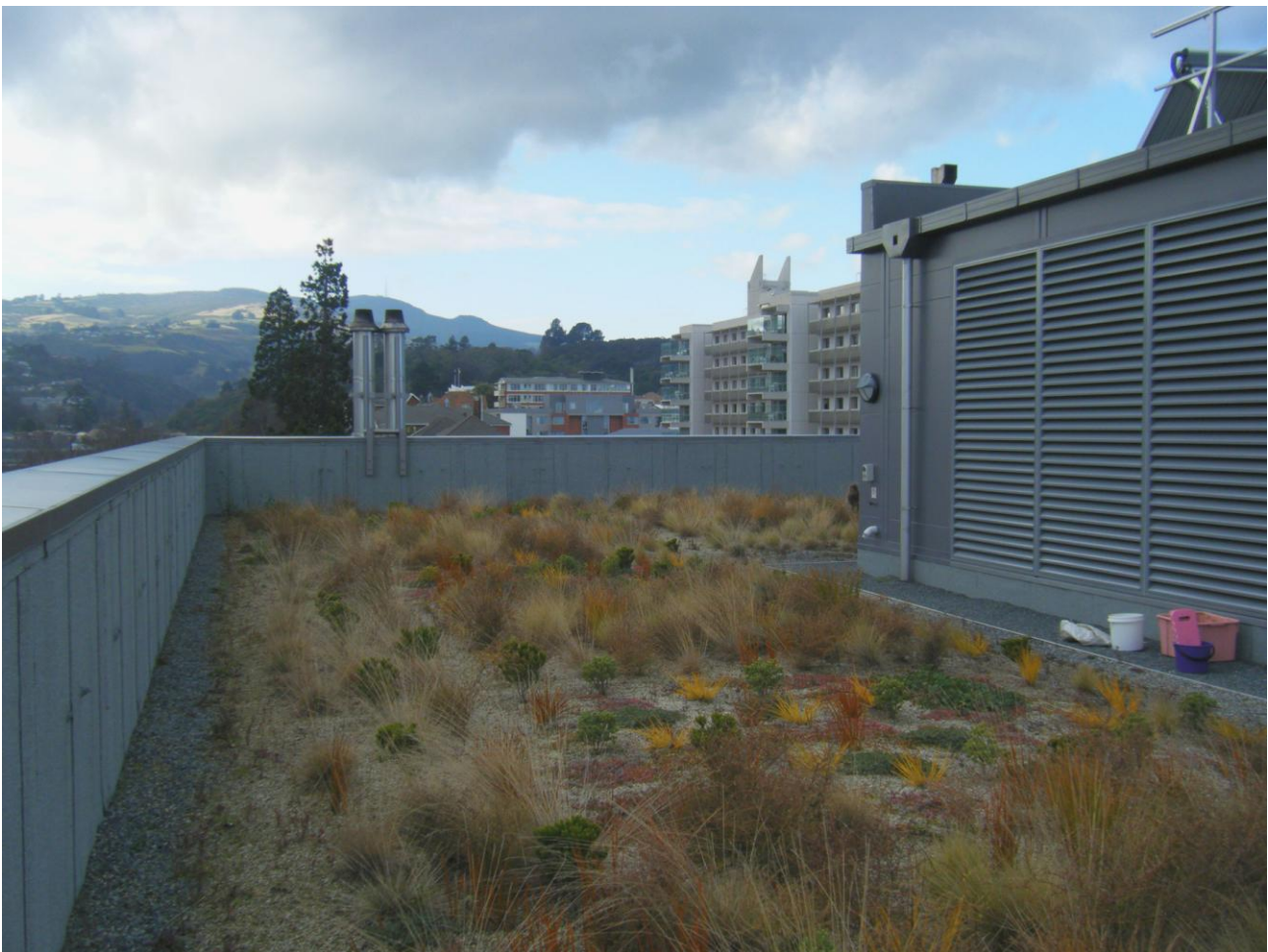
The green roof on top of Otago University's William James Psychology building. Photo by Janice Lord.
